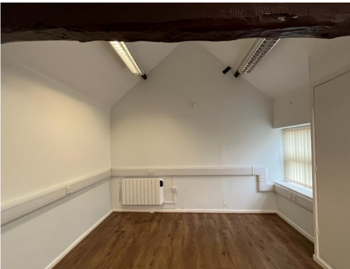
East Wall Internal
